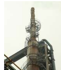
Mahong Plant's desulfurization tower
