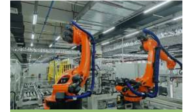
Intelligent production line of Chongqing Ganfeng in the New Lithium Battery Technology Industrial Park
